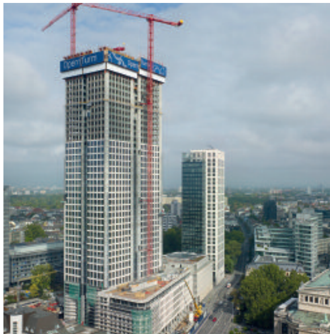
The Frankfurt OpernTurm during construction
