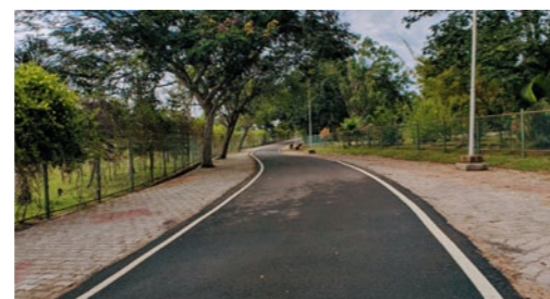
Asphalt road surface
