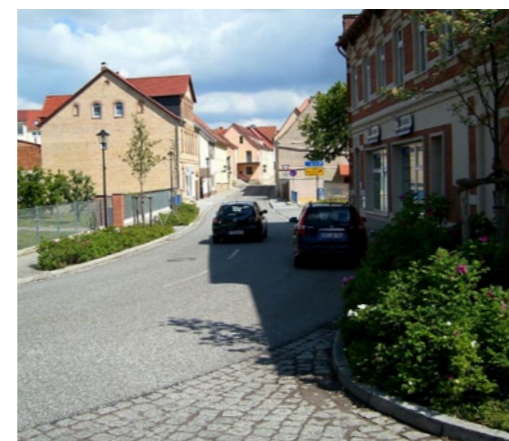
Asphalt with transition to natural stone sets
